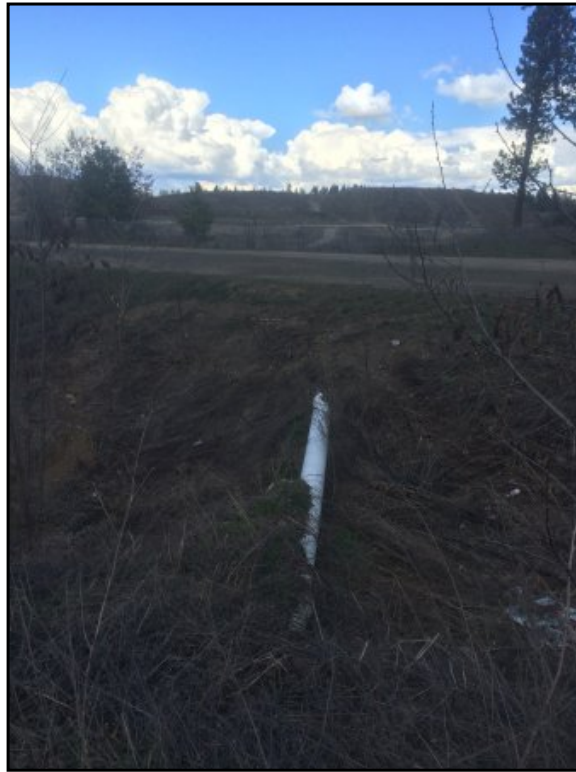
Zone 2 - Pond pipe
