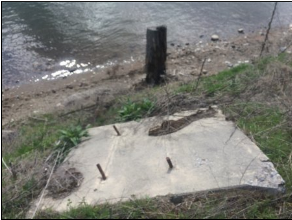
Zone 2 - concrete near shoreline. Potential bridge area
